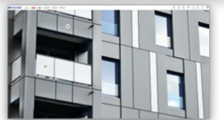
Balconies and parapets
